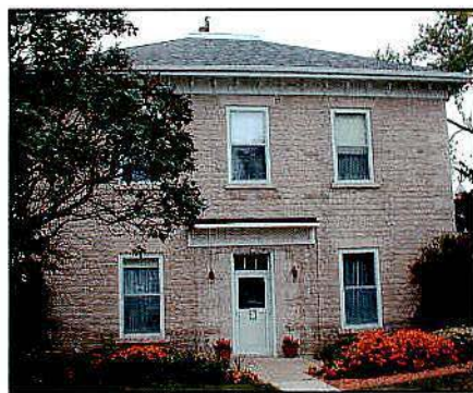
Still in use is the Rectory built by Fr. Daems
